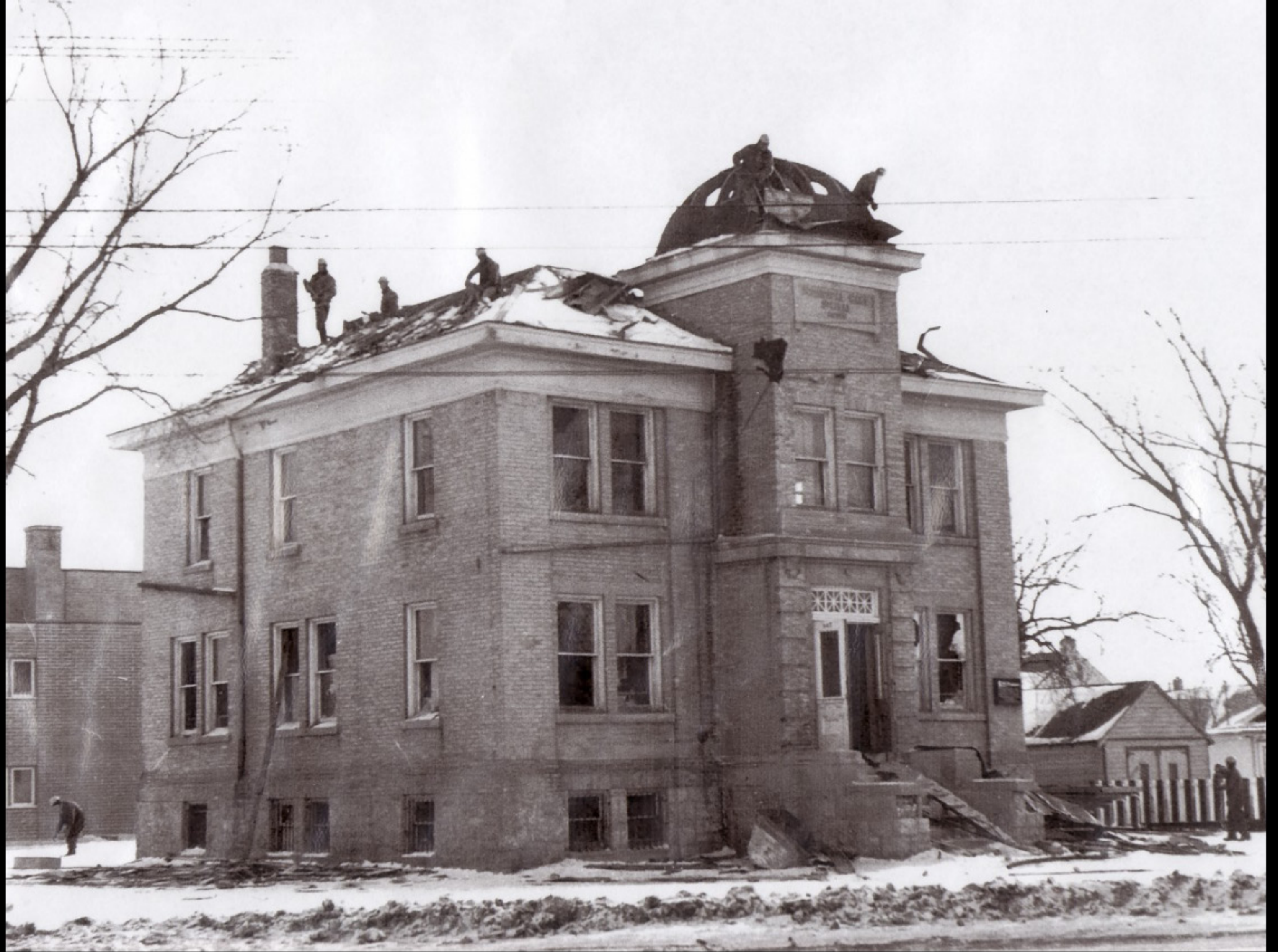
Building of Norberry Annex - Fernwood School
